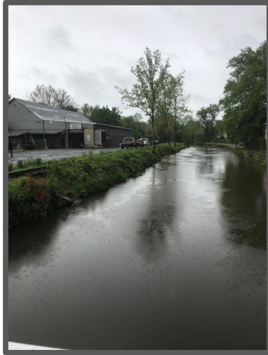
Figure 1 Photo of the Canal embankment post routine tree maintenance in Lambertville near Finkles.
